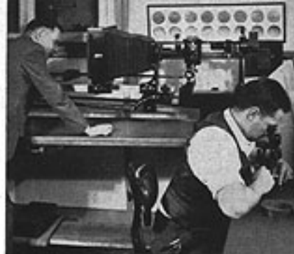
Making micro-photograph of steel.
